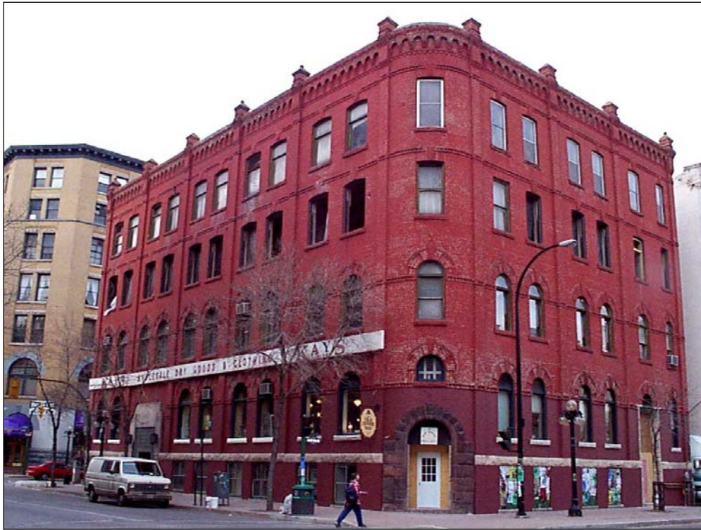
245 McDERMOT AVENUE – STOVEL BLOCK (KAY BUILDING)
