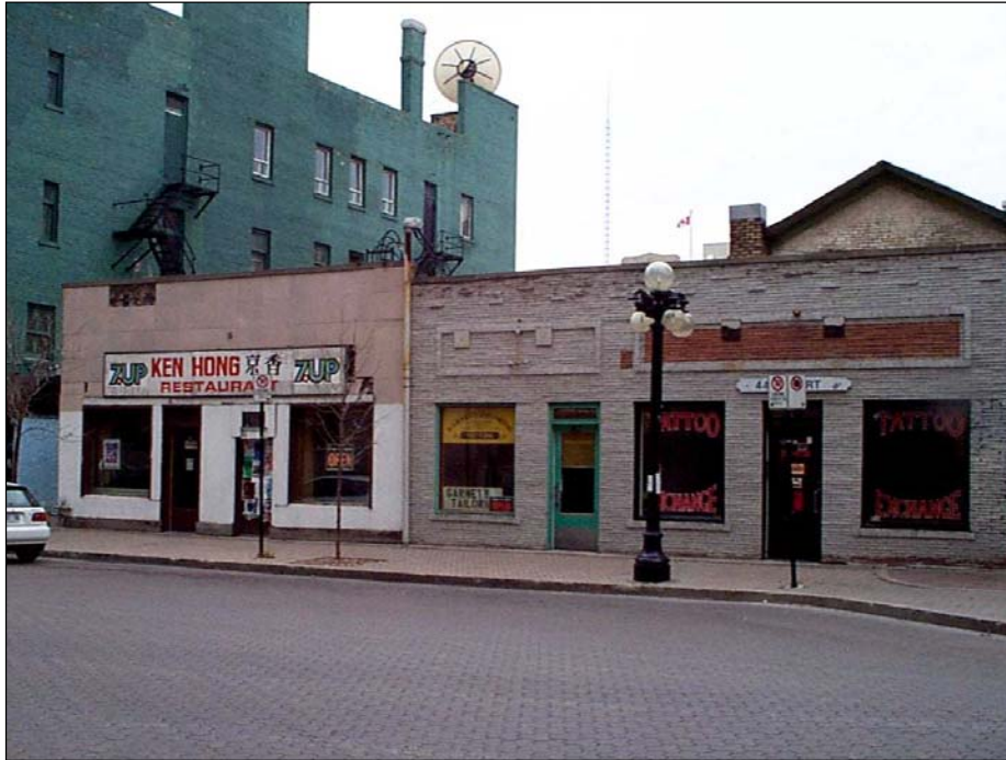
38 and 42 ALBERT STREET – ALBERT STREET BUSINESS BLOCK (38/42/44 ALBERT STREET)
