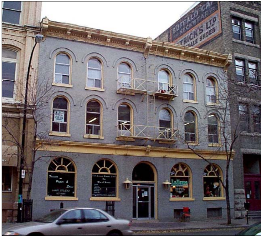
246 McDERMOT AVENUE – THOMSON-CODVILLE BUILDING (SURES BUILDING)
