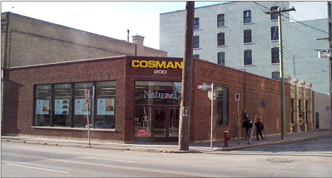
200 PRINCESS STREET – TORONTO HIDE & WOOL COMPANY BUILDING
