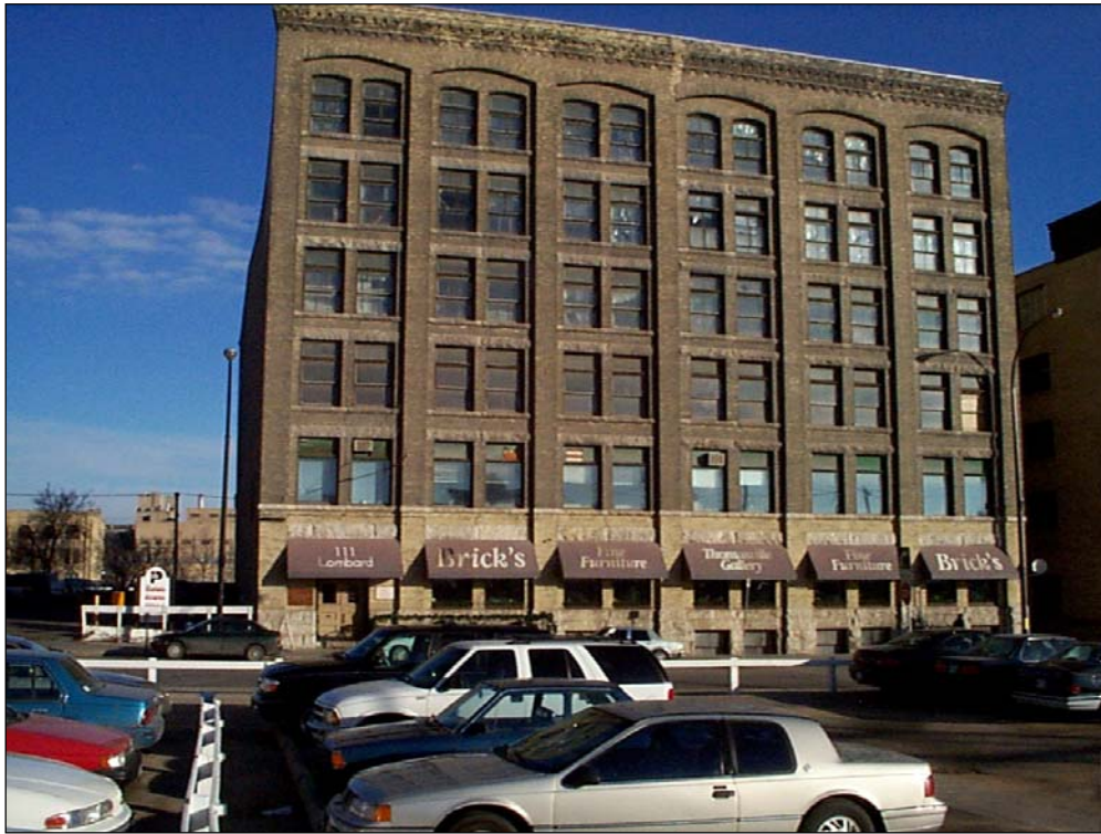
111 LOMBARD AVENUE – GAYLORD BLOCK (KEMP BUILDING) (110 McDERMOT AVENUE)
