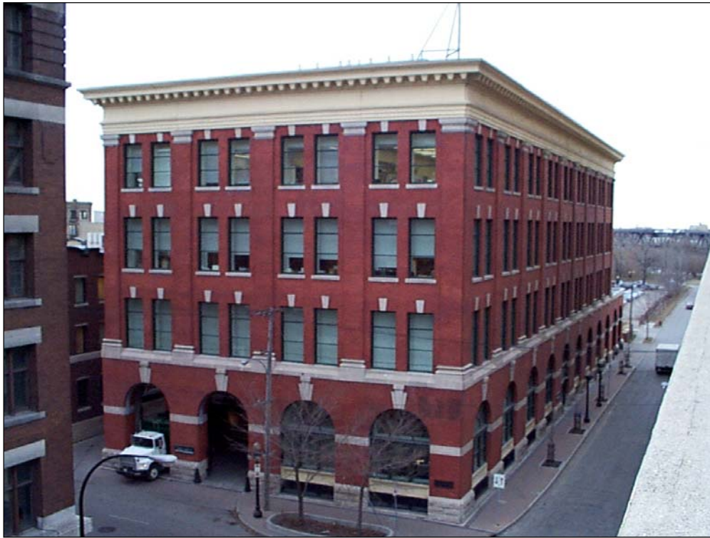
145 McDERMOT AVENUE – CUSTOMS EXAMINING WAREHOUSE
