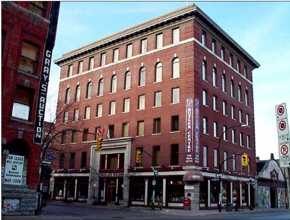
283 BANNATYNE AVENUE – TRAVELLERS BUILDING
