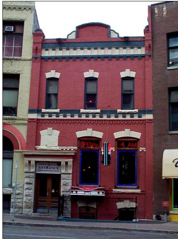
177 McDERMOT AVENUE – T.W. TAYLOR BUILDING
