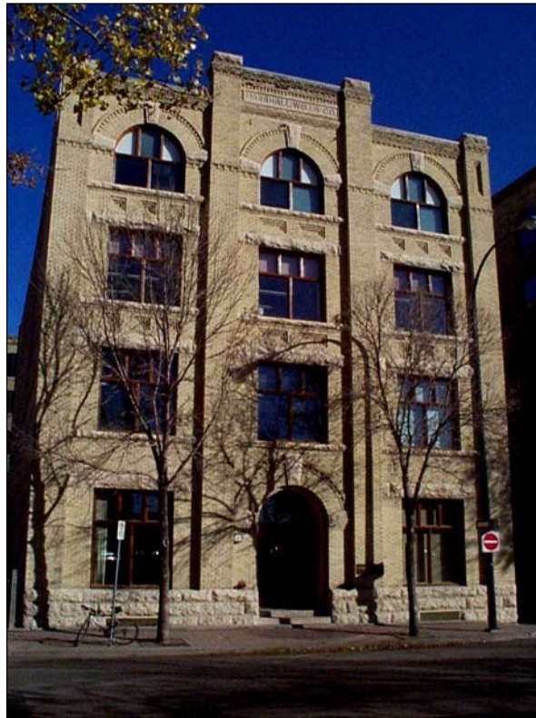
123 BANNATYNE AVENUE – MARSHALL-WELLS BUILDING
