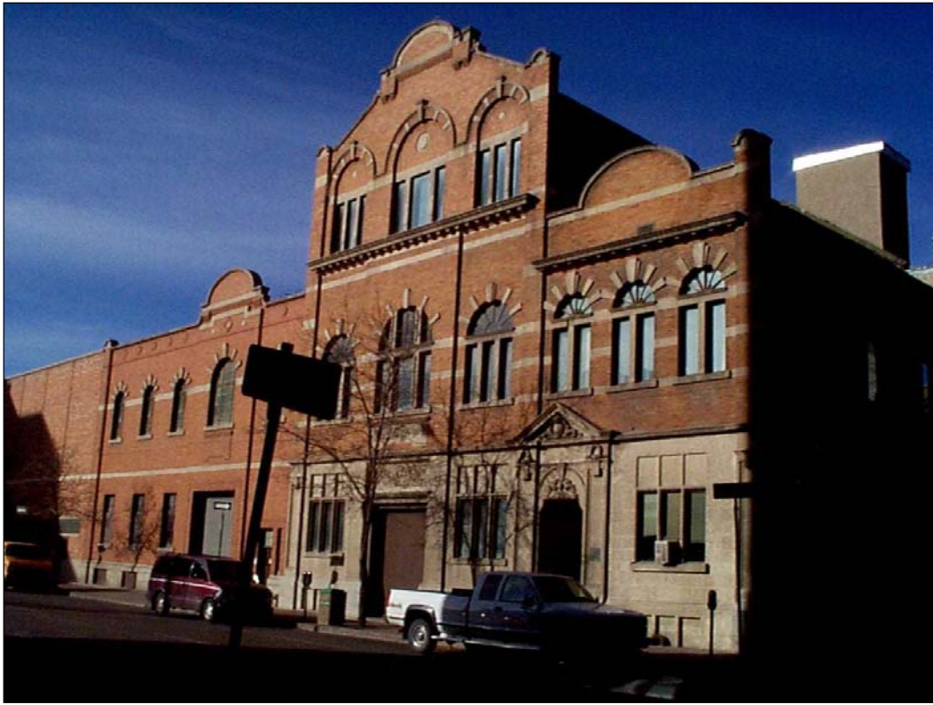
54 KING STREET – WINNIPEG HYDRO SUB-STATION NO. 1 (48/54 KING STREET & 55 PRINCESS STREET)
