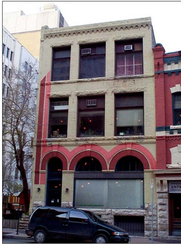
179 McDERMOT AVENUE – W.F. ALLOWAY BUILDING
