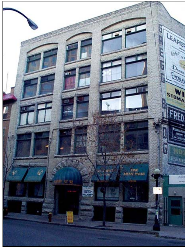
52 ALBERT STREET – GREGG BUILDING (52/54/56 ALBERT STREET)
