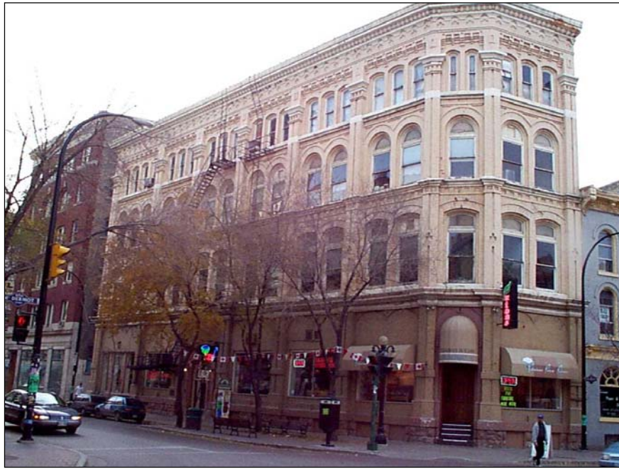
70 ALBERT STREET – TELEGRAM BUILDING (SURES BLOCK) (68/70 ALBERT STREET)
