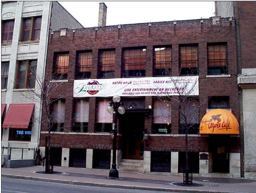
171 McDERMOT AVENUE – DAWSON RICHARDSON BUILDING
