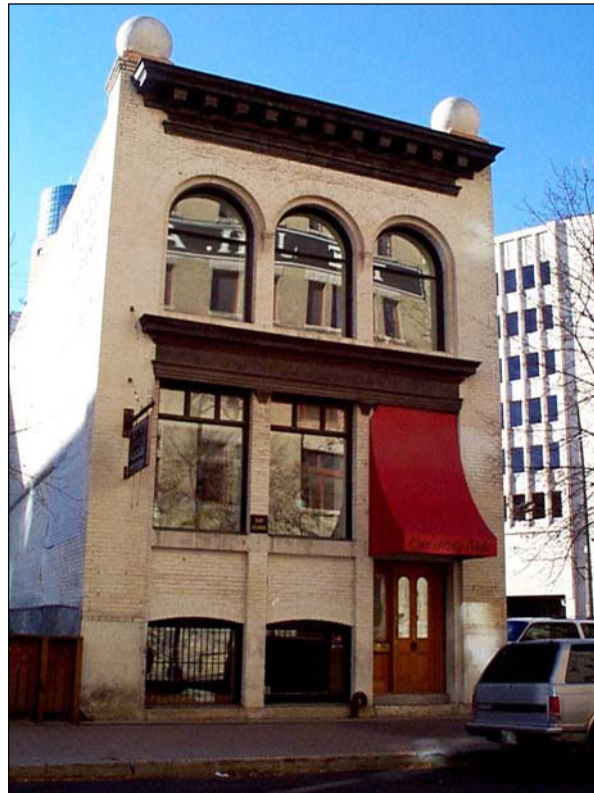
168 BANNATYNE AVENUE – FRANKLIN PRESS BUILDING (CHATFIELD DISTRIBUTORS)
