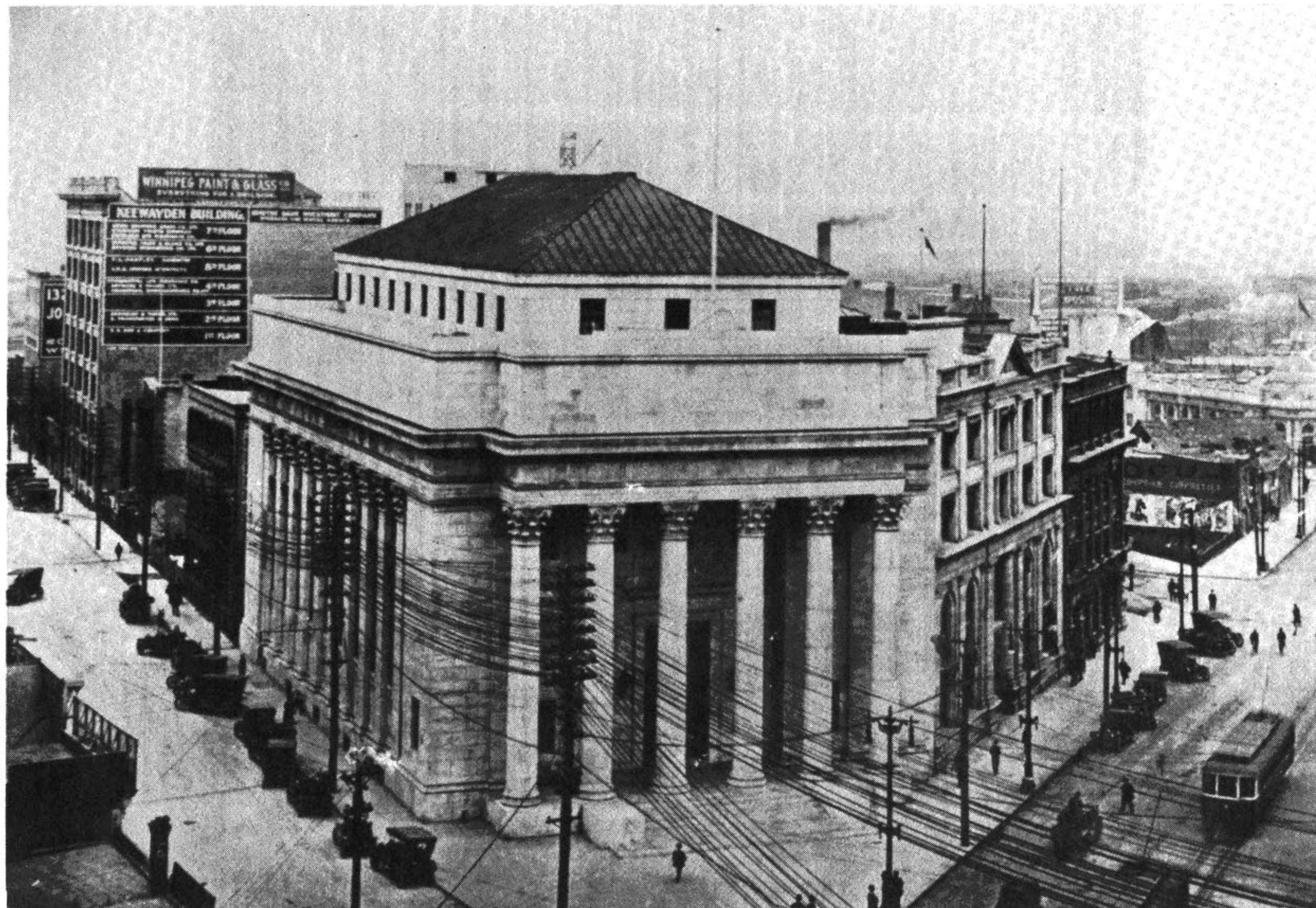
A 1914 illustration graphically illustrates the Bank of Montreal's prominent position at the intersection of Portage and Main.
