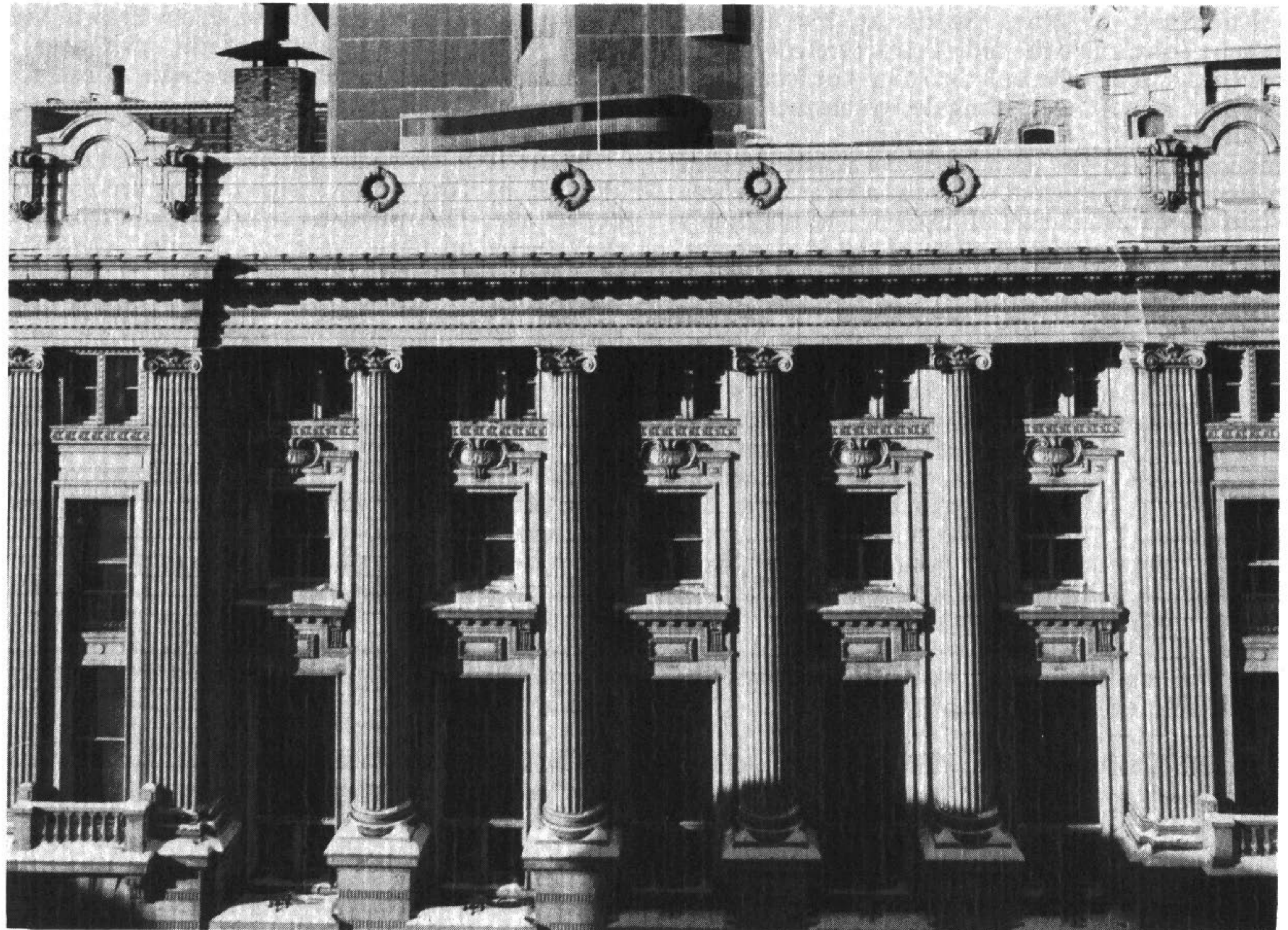
The intricate terra cotta of the east facade. The terra cotta was shipped custom-made from England.
