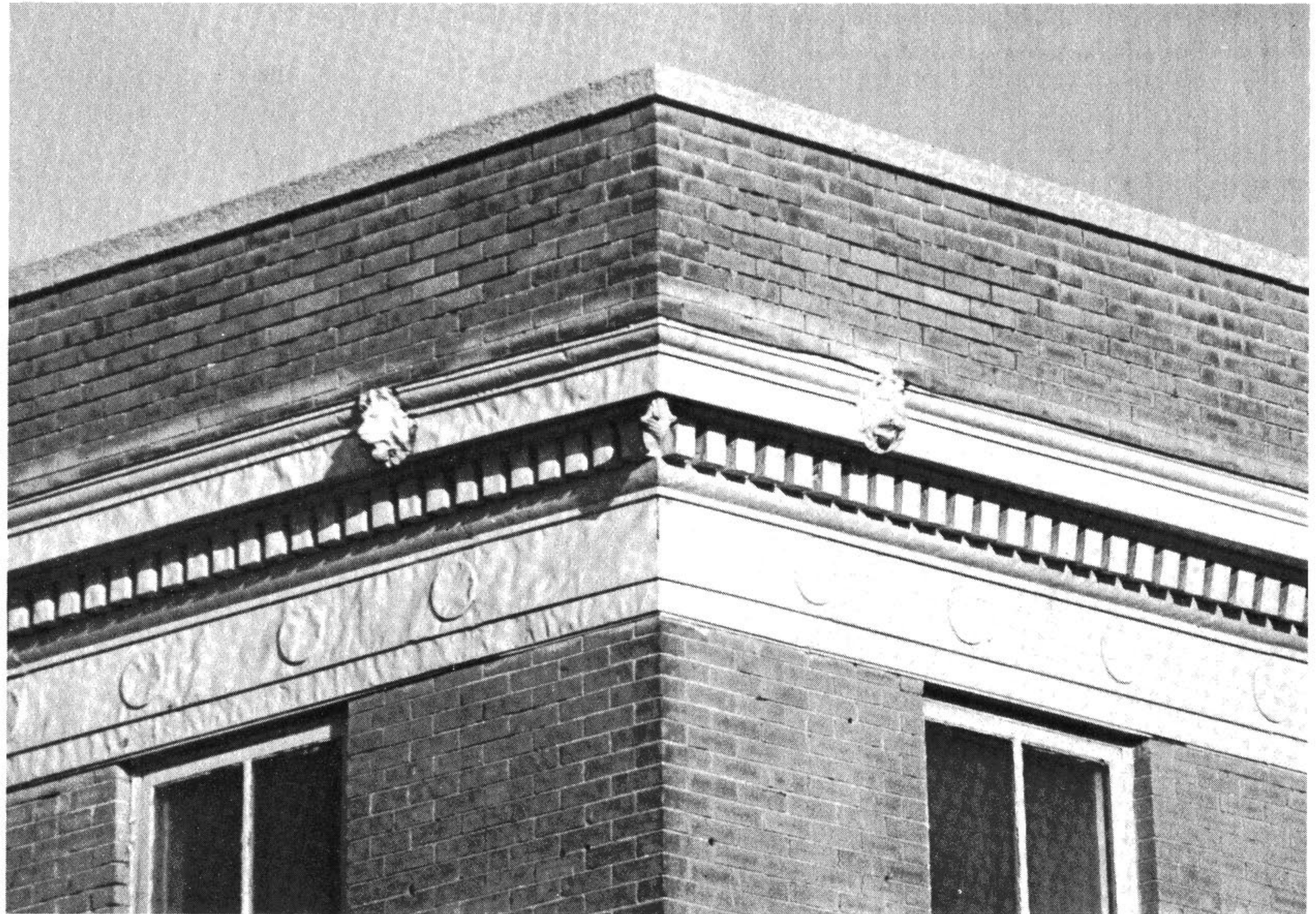
Detail of galvanized iron cornice with brick parapet.
