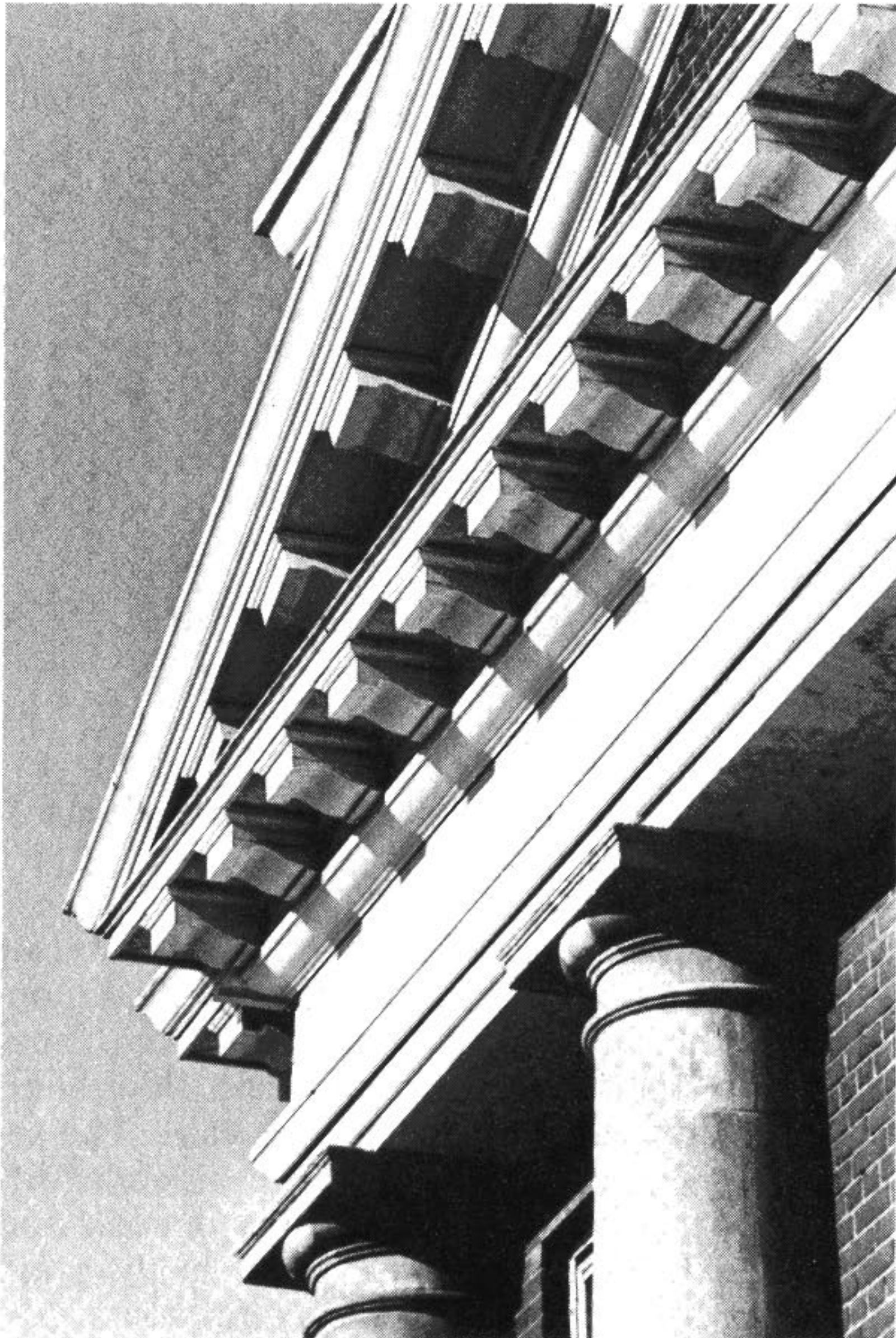
Much of the exterior ornamentation of the bank is prefabricated.
