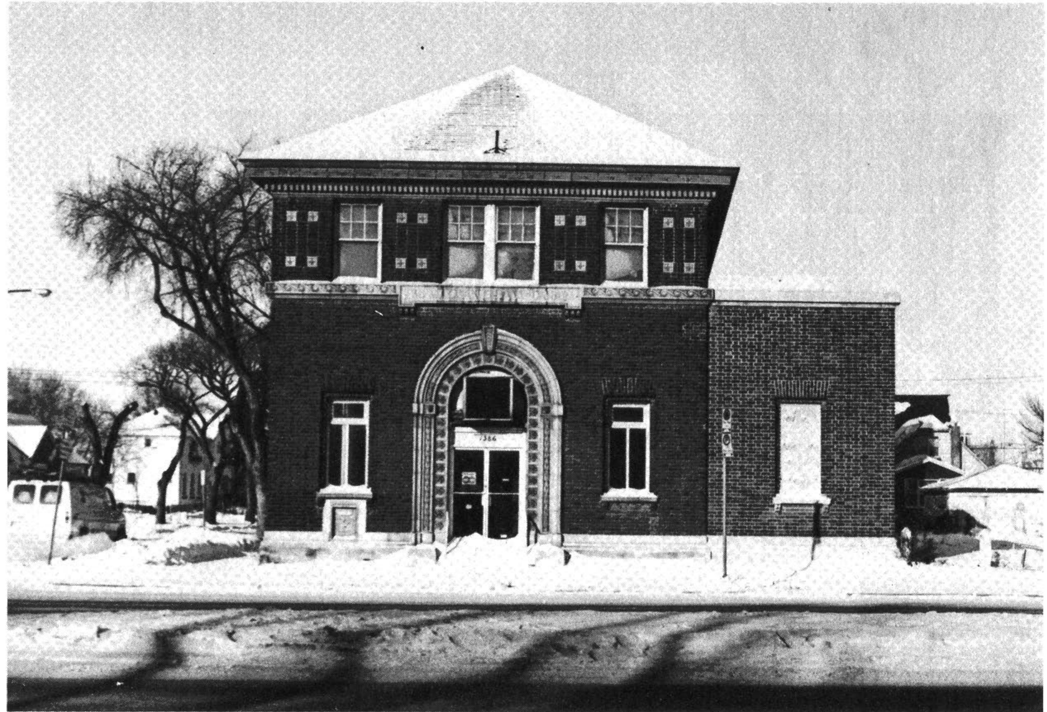
Merchants Bank, Main Street facade.
