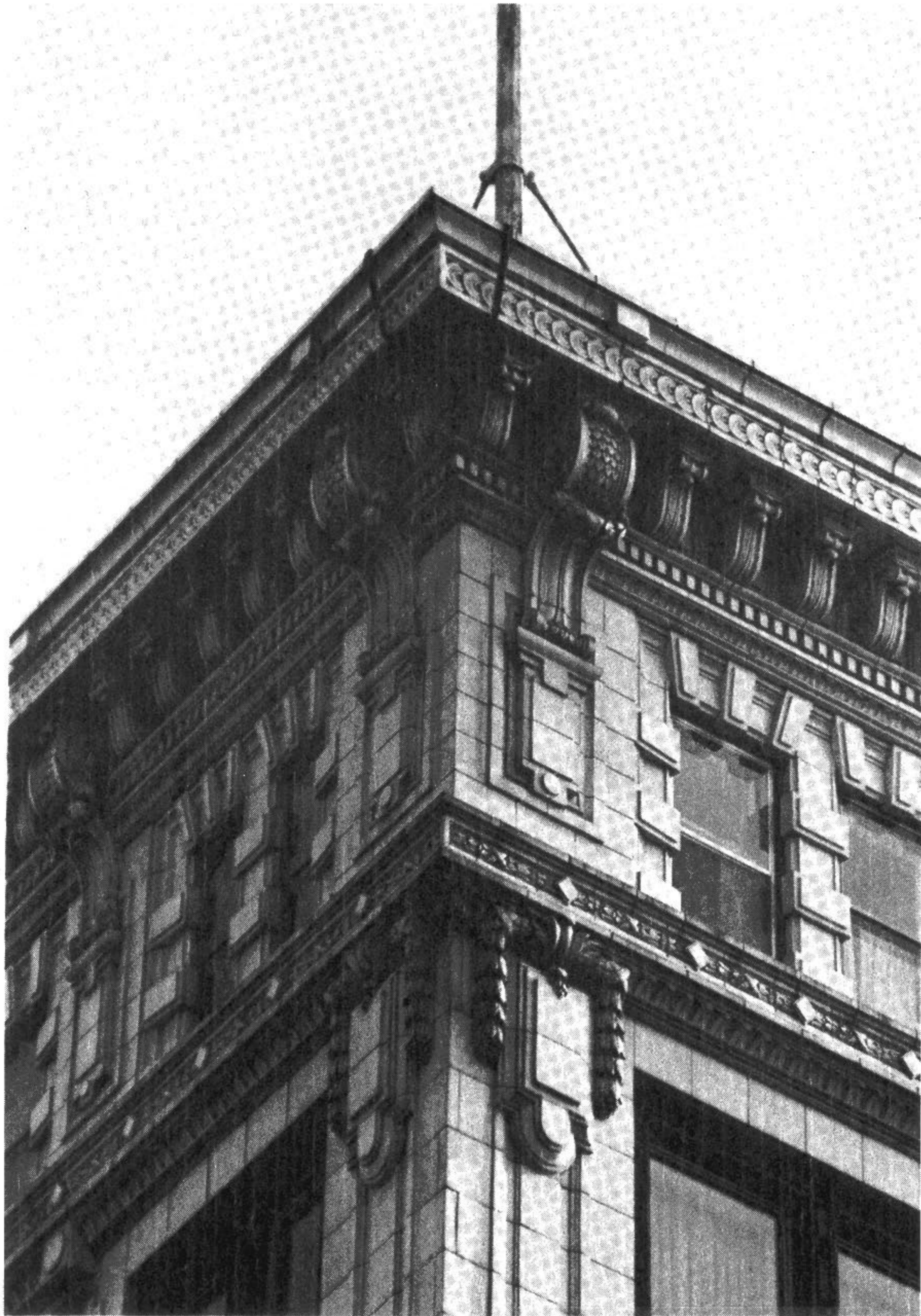
Cornice detail, Boyd Building
