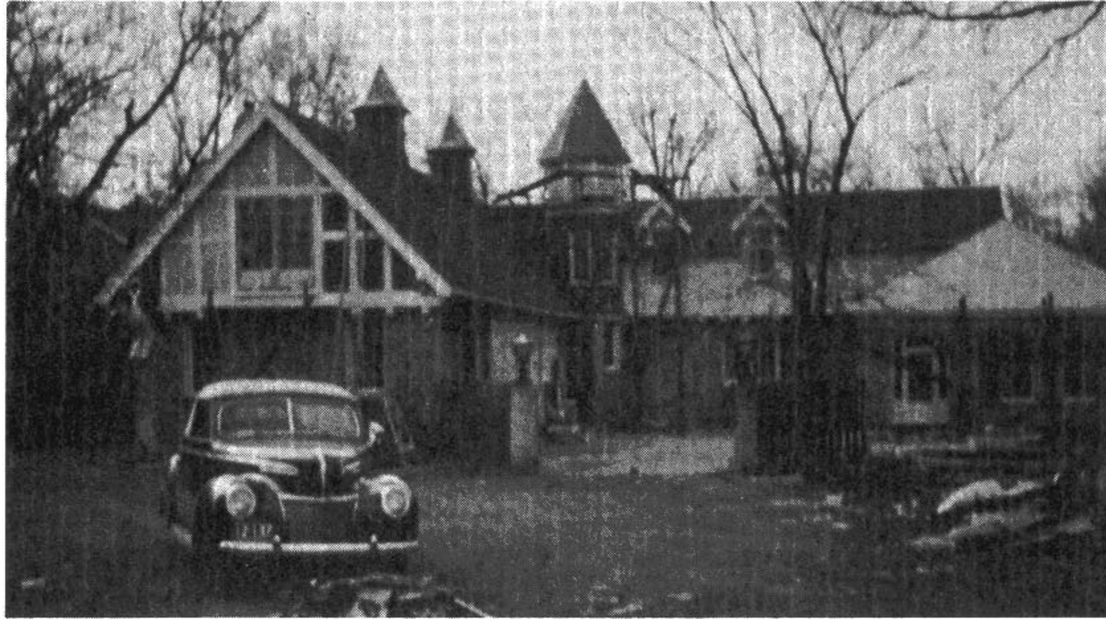
Demolition and Construction 1940
