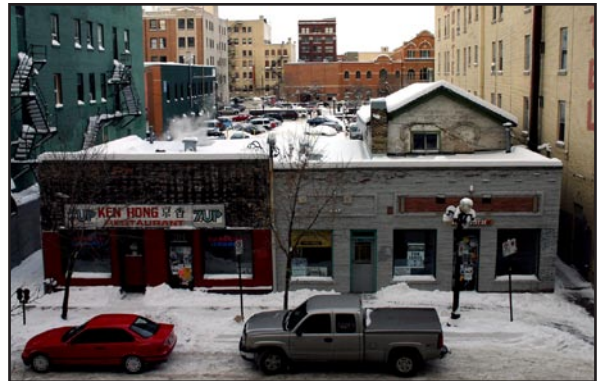
Front of the Albert Block and J.O. LeCappellain House, 38-44½ Albert Street
