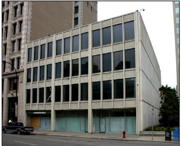
Electric Railway Chambers Annex, 219 Notre Dame Avenue
