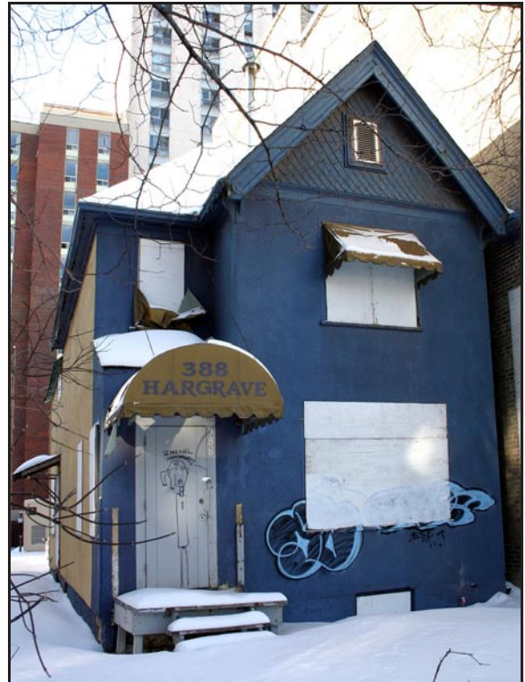
Cole House, 388 Hargrave Street
