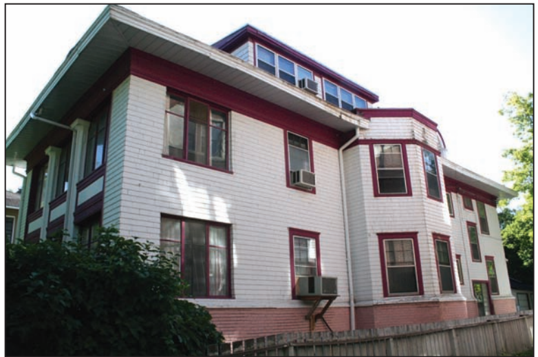
Peterson Duplex, 260 Wellington Crescent
