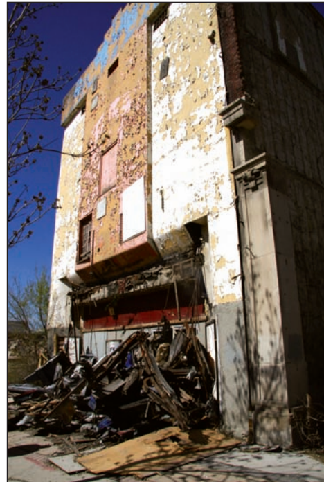
The Rex Theatre, 646 Main Street, shortly before its demolition, May 2008
