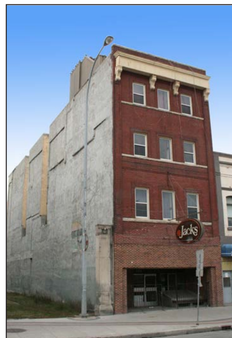
Jack's Place, 652 Main Street, shortly before its 2008 demolition
