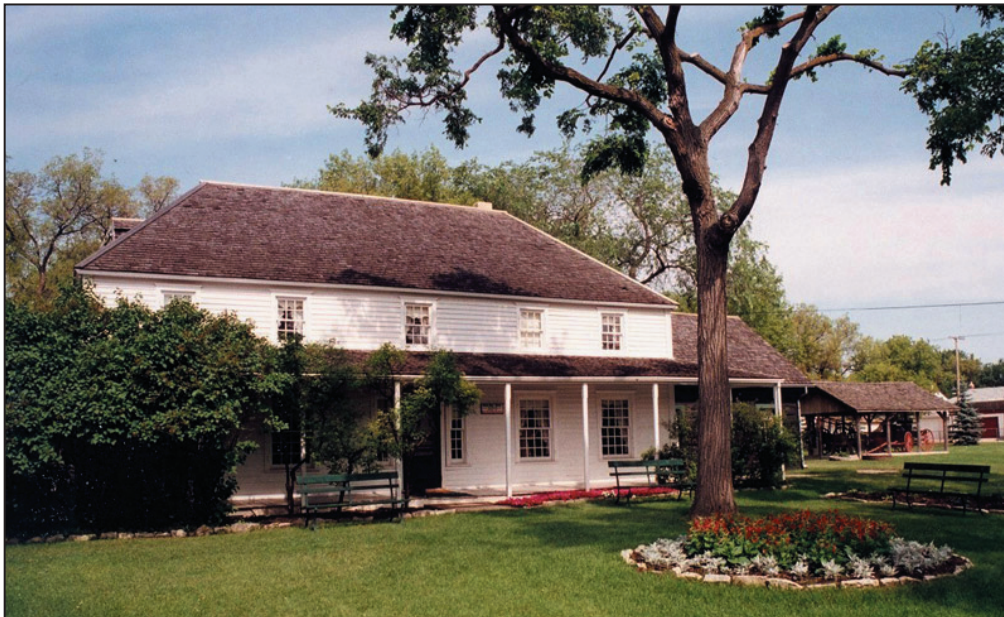
Seven Oaks House Museum, 115 Rupertsland Avenue
