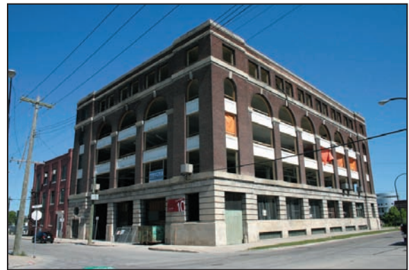
Renovations being completed on the 1913 portion of the Smart Bag Company Building
