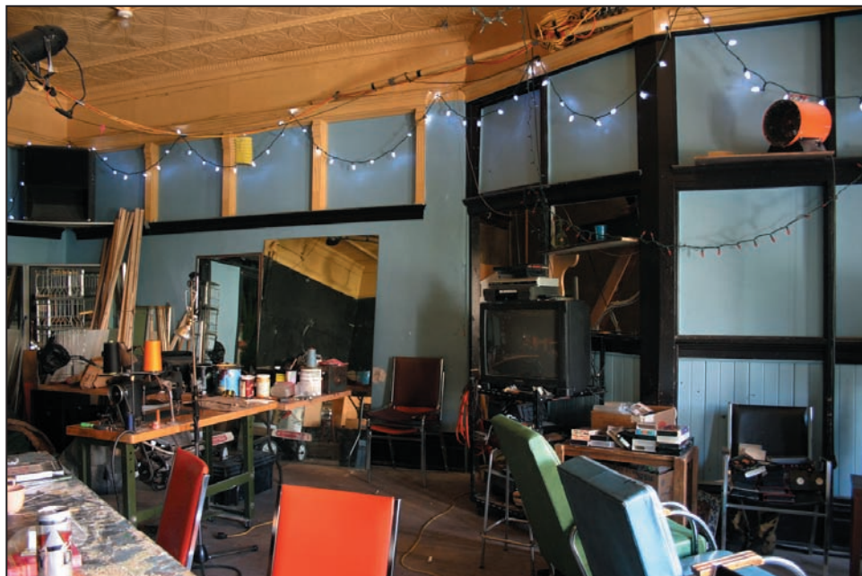
Part of the second floor with its original wood and glass partitioning and tin ceiling
