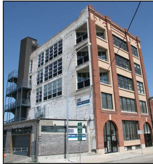
448 Hargrave Street, Clark Brothers Warehouse
