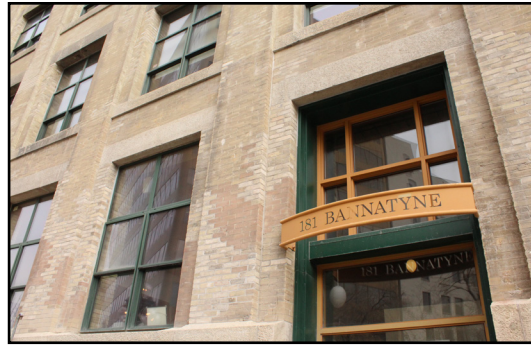
181 Bannatyne Avenue, Kilgour Block, repaired masonry on the front (south) façade
