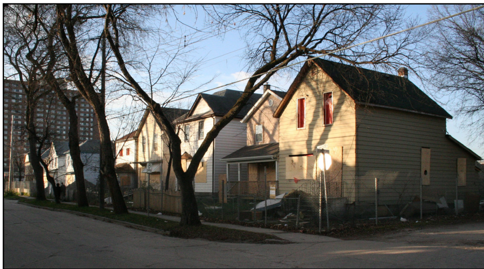
Neglected houses in the 300 block of Langside Street just prior to demolition, 2007
