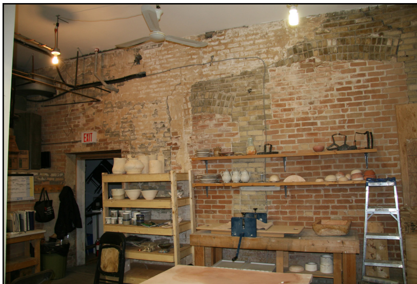
Interior brick wall on the main floor of the Corbett Block
