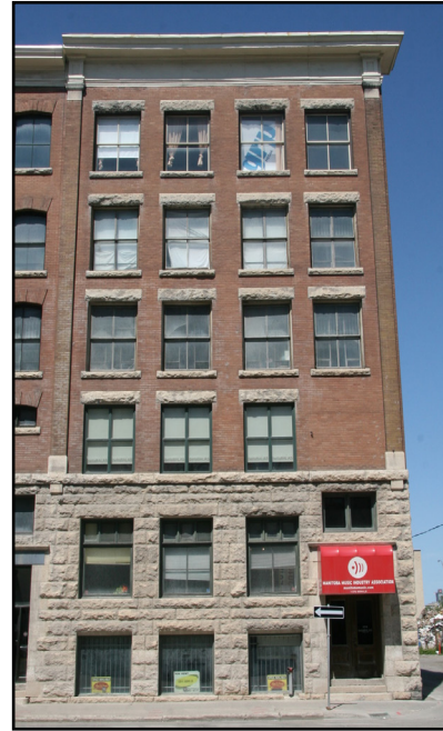
376 Donald Street, Aldous Building
