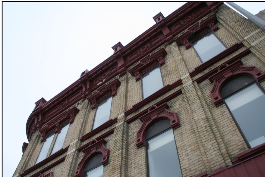
Part of the front façade of the Maycock Block, 586 Main Street
