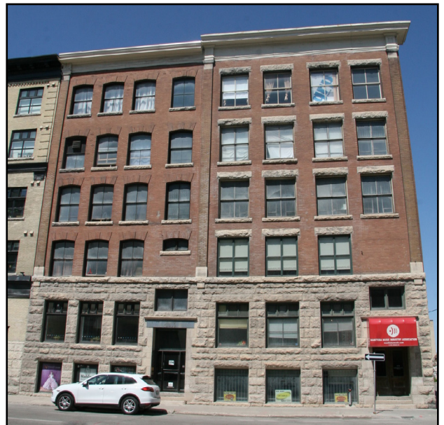
Aldous Building Annex (left) and Aldous Building (right)
