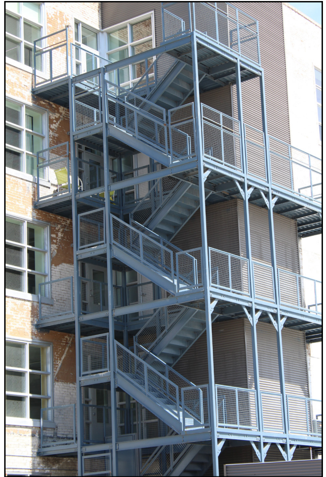
New rear staircase/balcony system for the renovated Clark Brothers Warehouse
