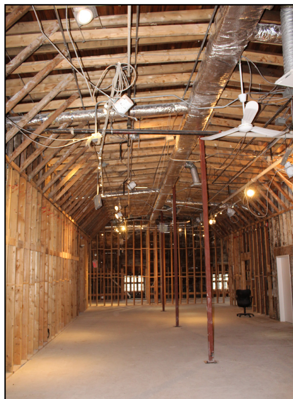
55 Pavilion Crescent, Assiniboine Park Pavilion, gutted 3rd floor
