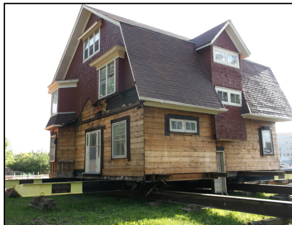
51 Balmoral Street, Milner Residence, raised off its original foundation, July 2016
