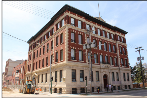
474 Hargrave Street, Manitoba Telephone System – Garry Exchange
