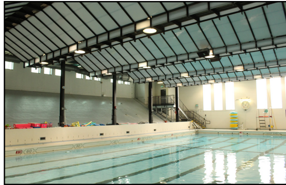
381 Sherbrook Street, Sherbrook Pool with its newly renovated interior
