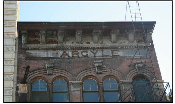
Detail of the upper floors, Garry Street façade, Argyle Block
