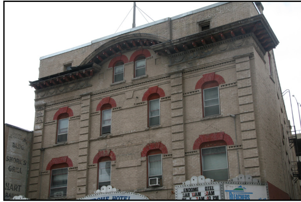
The Vendome Hotel with its ornate metal cornice intact, July 2015.
