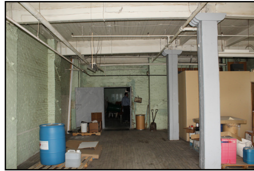
Second floor of the 1898 section of the Thomas Black Building
