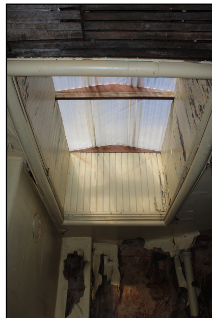
Skylight in the Guest Block
