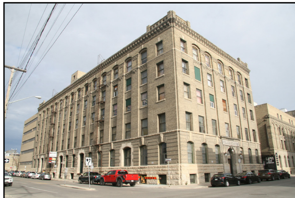
317 McDermot Avenue, Miller, Morse and Company Building
