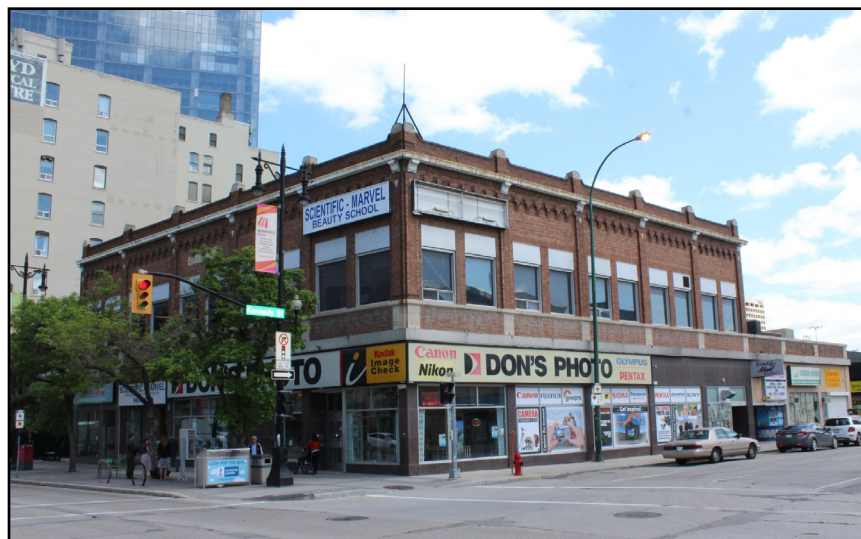
410 Portage Avenue, Bradburn Block
