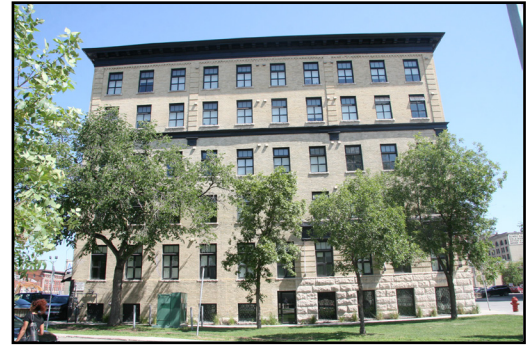
South façade of the Bell Block
