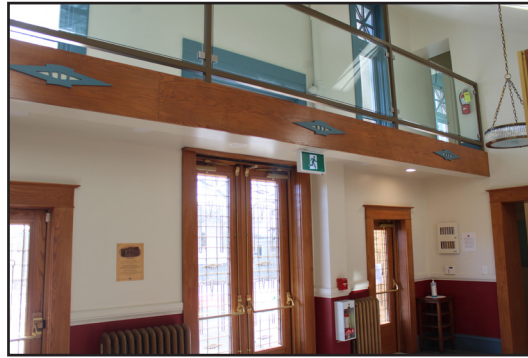
Ukrainian Labor Temple, 591 Pritchard Avenue, restored entrance lobby with new second floor walkway, 2021. (M. Peterson)
