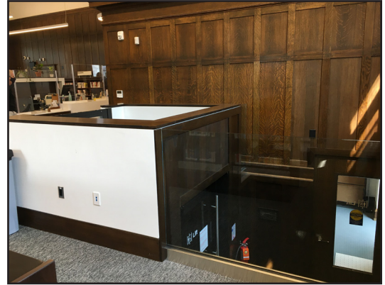
Cornish Library, 20 West Gate, new lift in original library, 2021. (R. Ricci)
