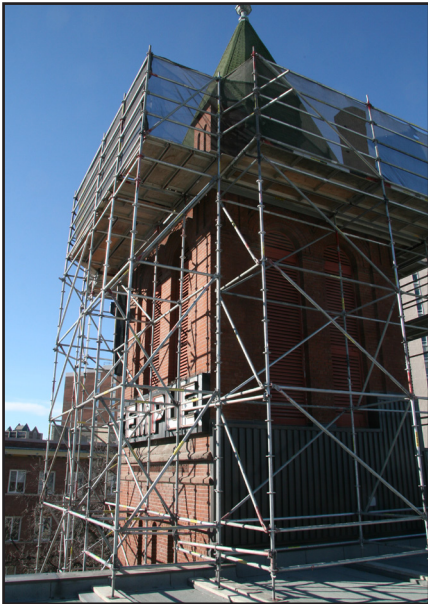
Scaffolding on the tower at Calvary Temple, 400 Hargrave Street, 2021. (G. Menzies)
