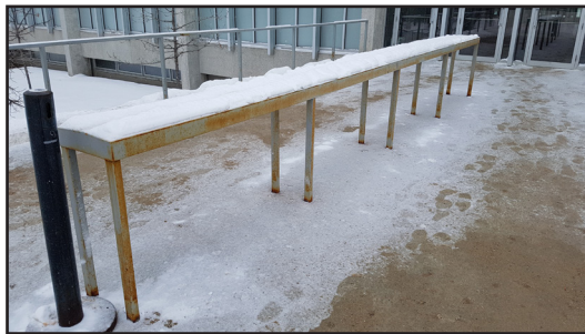
J.A. Russell Building, University of Manitoba, 83 Dafoe Road, restoration underway, 2021. (G. Menzies)
