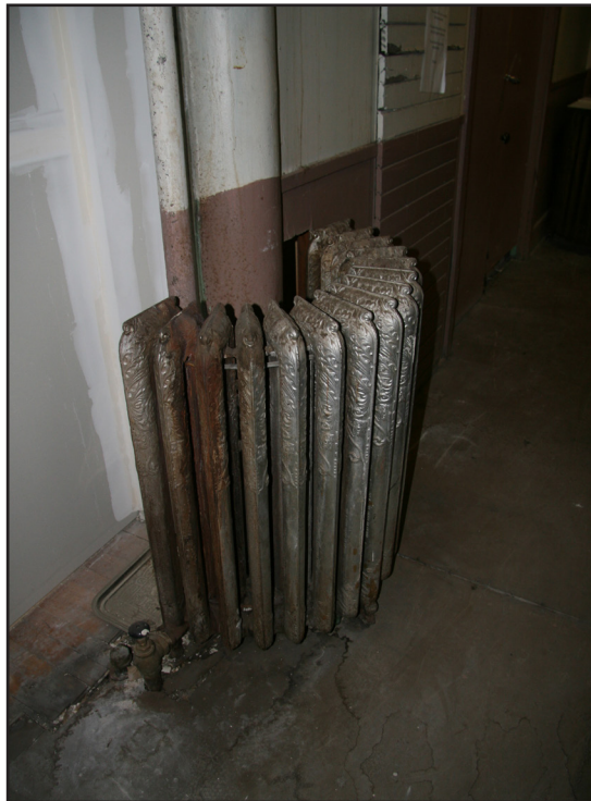
This unusual curved radiator is found on the third floor of the Stobart and Sons (Bedford) Building, 275 McDermot Avenue. (M. Peterson)
