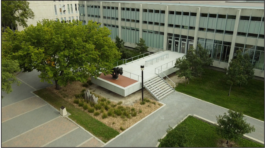
J.A. Russell Building, University of Manitoba, 83 Dafoe Road, restoration completed, 2021. (University of Manitoba)
