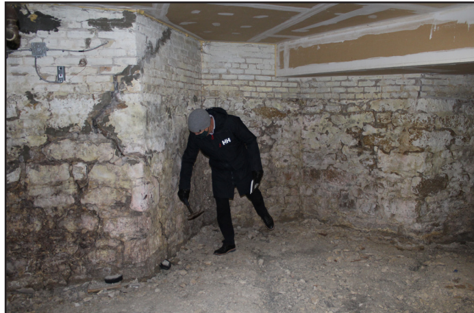
Committee member J. Wells, observing a basement foundation. (M. Peterson)
