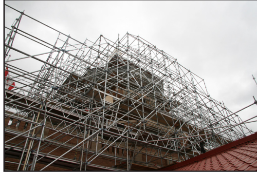
Administration Building, University of Manitoba, 66 Chancellors Circle, scaffolding on the cupola, 2021. (G. Menzies)
