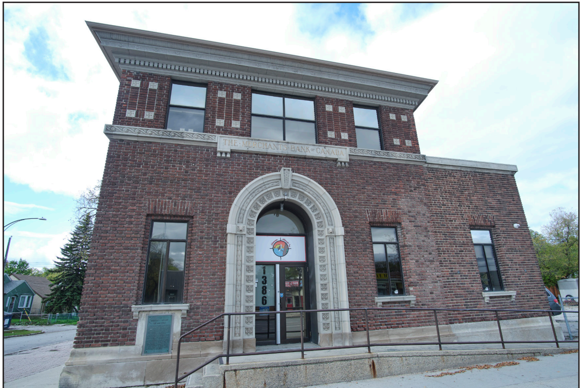
Built as a Merchants Bank branch in the North End in 1913, this building at 1386 Main Street is now used Shawenim Abinoojii Inc., offering support for people in the Southeast Tribal Region. (G. Cline)
