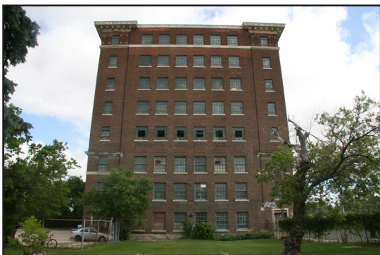
90 Annabella Street, J.R. Watkins Company Factory and Warehouse, south façade, 2021. (G. Menzies)
