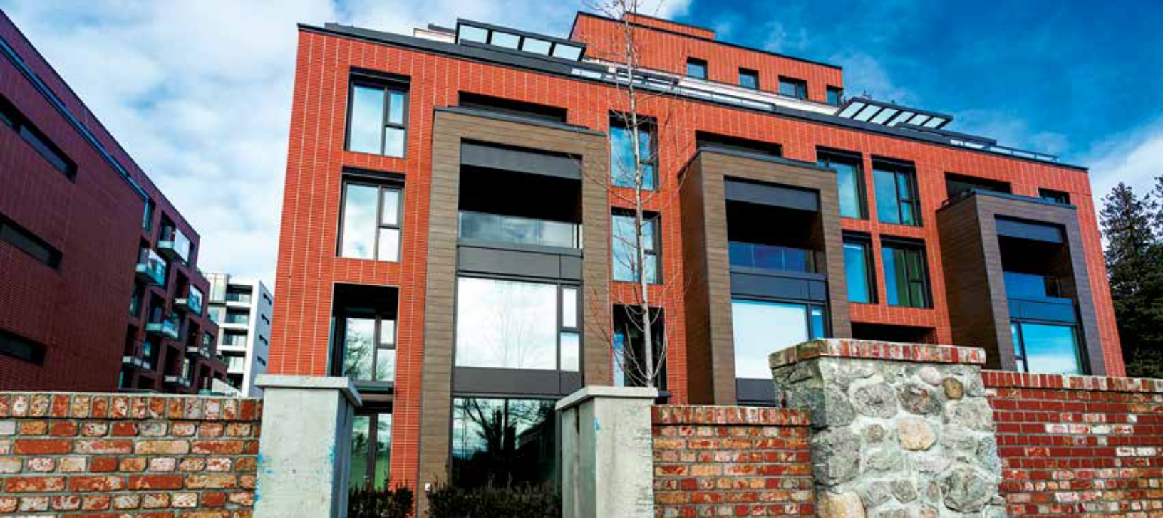
Multi-unit dwelling that incorporates high-quality materials and steps back taller portions of the building.
