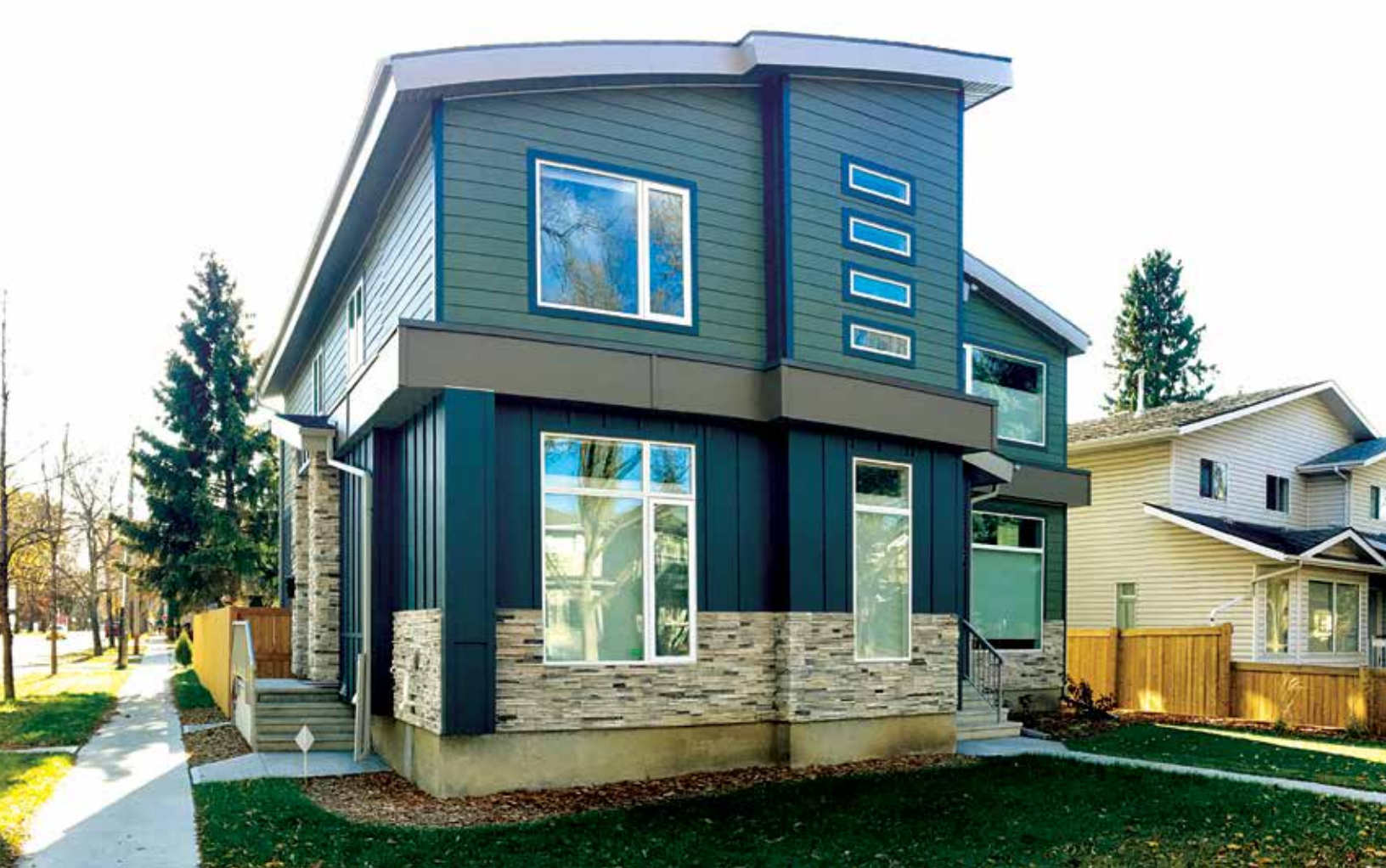
Triplex on corner lot with entrances facing both streets and building setbacks that align with adjacent dwelling.
