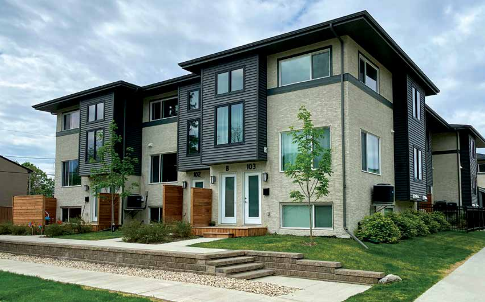
An example of a townhouse dwelling demonstrating articulation through recesses and projections.
