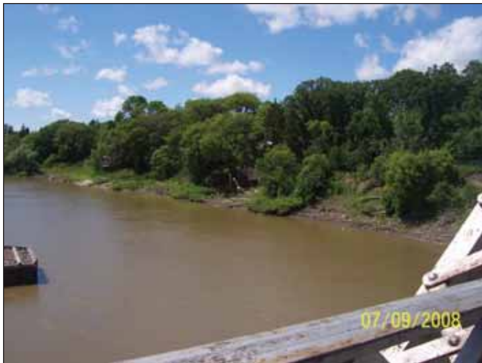
Photo 4 – Looking upstream from Elm Park Foot Bridge at ongoing riverbank instability.
