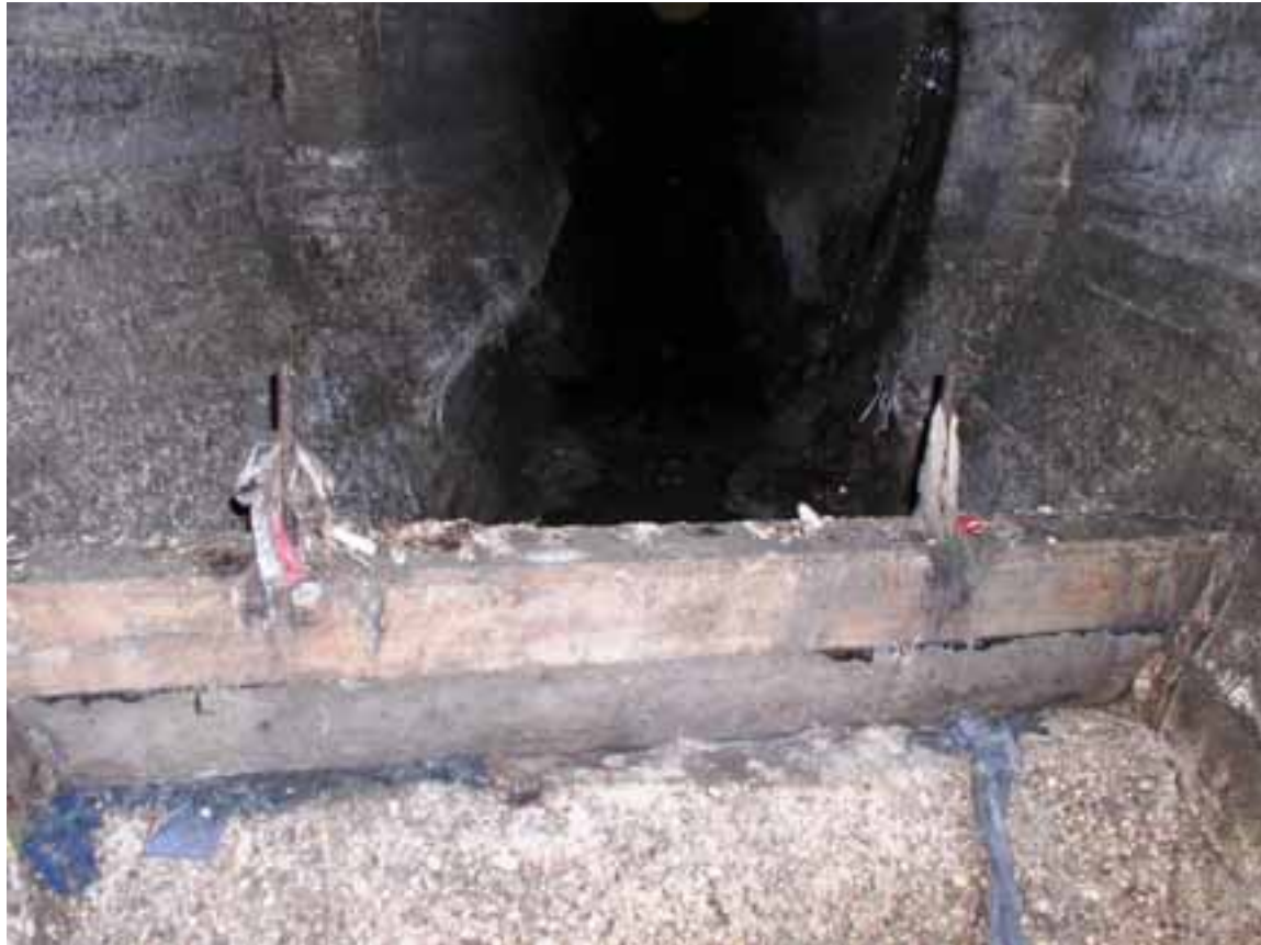
Photo 12-1: Cockburn Fixed Weir With Stop Log Additions
