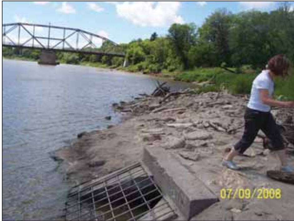
Photo 3 – Outlet of existing high level outfall at Cockburn.
