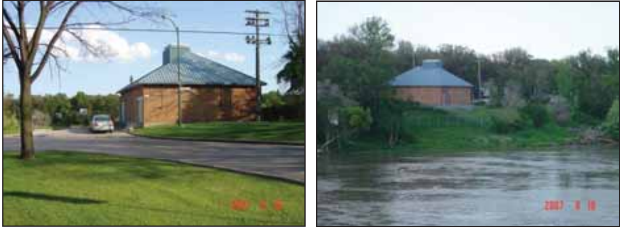
Photo 11-1: Cockburn Flood Pumping Station
